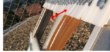
Figure 2: Clamps made of ultra-high molecular weight polyethylene
